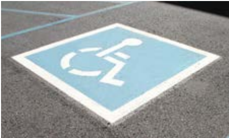
ADA "Blue-Paint" Access
